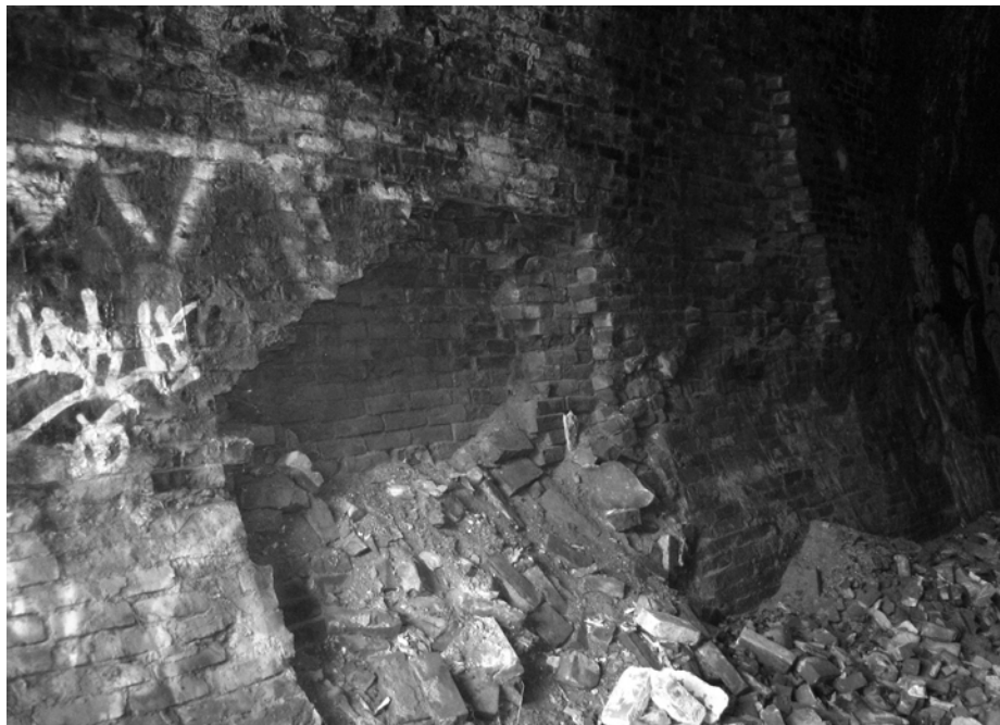
Figure 3. Deteriorated brick lining in 2007
