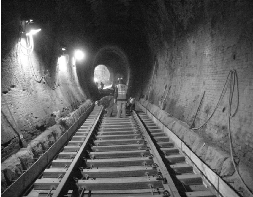
Figure 6. Rigid track structure being assembled
